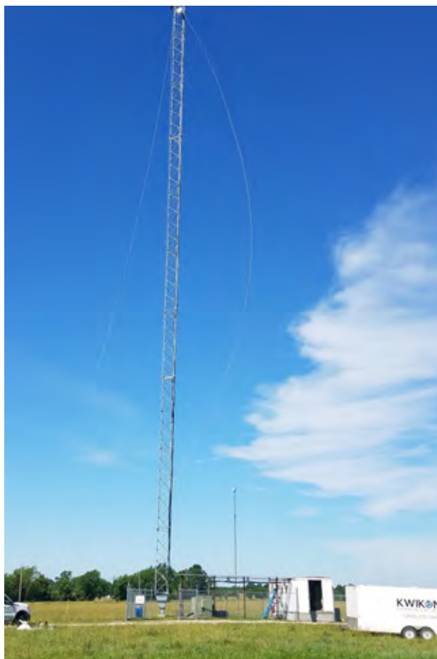
Even the fastest wireless tech needs fiber at the tower to achieve speeds of 100 Mbps or more. Source: Kwikom.
